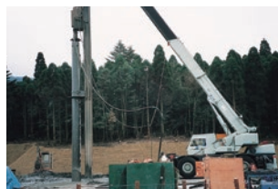
Geothermal, Oil Well Surface drilling down to 50m in depth for geothermal and oil well.
